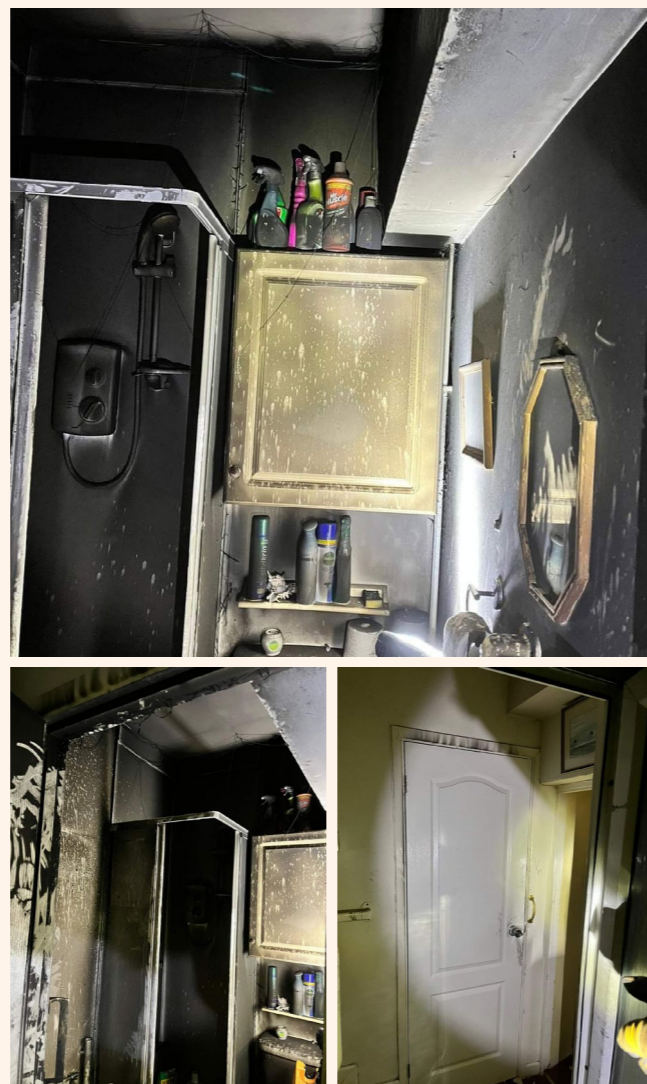
Pictured above: A fire caused by an extraction fan. The occupants kept their bathroom fire door closed, and the fire was limited to that room until the Fire Service arrived.
